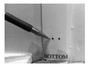
3) Puncture the **BLACK CIRCLES (Figure 2)** and mark with a pencil the 4 screw locations, at the bottom and top of the template, in the center of the circles. Remove the template and where you just marked with pencil drill with 5/64" drill bit a pilot hole for screws **(B)**.
